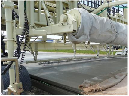
The longitudinal tining kit uses the same hydraulic controls as the transverse tine cart and mounts to the adjustable transverse cart track. Tine rakes can be hydraulically raised or lowered. Longitudinal tining can be done concurrently with the curing operation.
