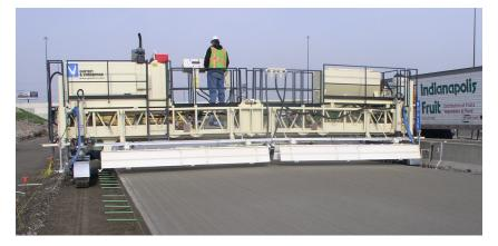
The TC1500 can be equipped with one or more crowning points that are hydraulically controlled from the Operator Console. Using optional sonic crowning sensors, the machine frame can be programmed to transition automatically in and out of crown in reference to the profile of the road surface.
