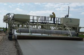
As an option, a Poly-Roll Attachment with manually adjustable support arms can be supplied for quick slab protection from rain. The support arms hinge up for transport. The roll is hydraulic motor powered for fast lay down and pick up of the polyethylene paper.
